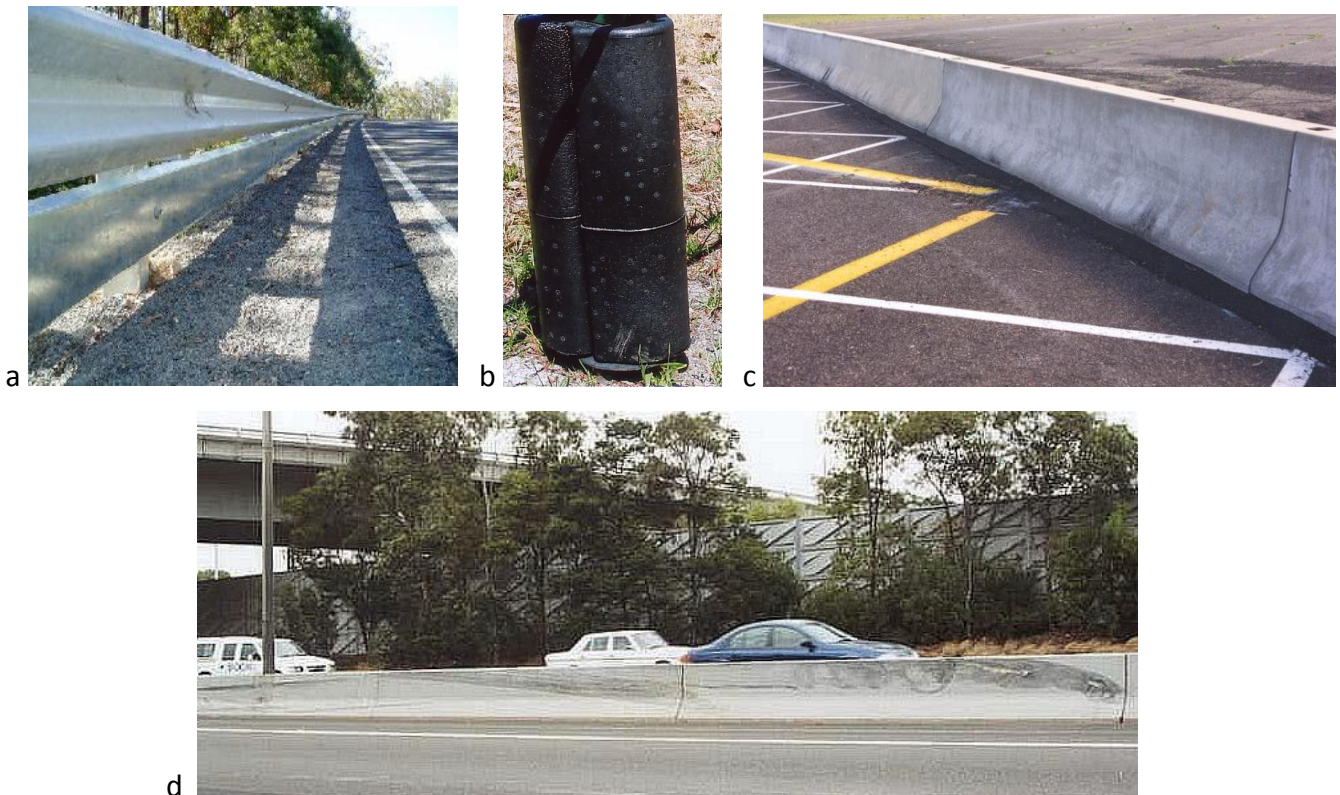
Figure 1: Examples of; a) steel rub-rail system, b) padded post protector and c) continuous concrete barrier d) wheel prints on concrete barrier showing evidence of vehicle launching
